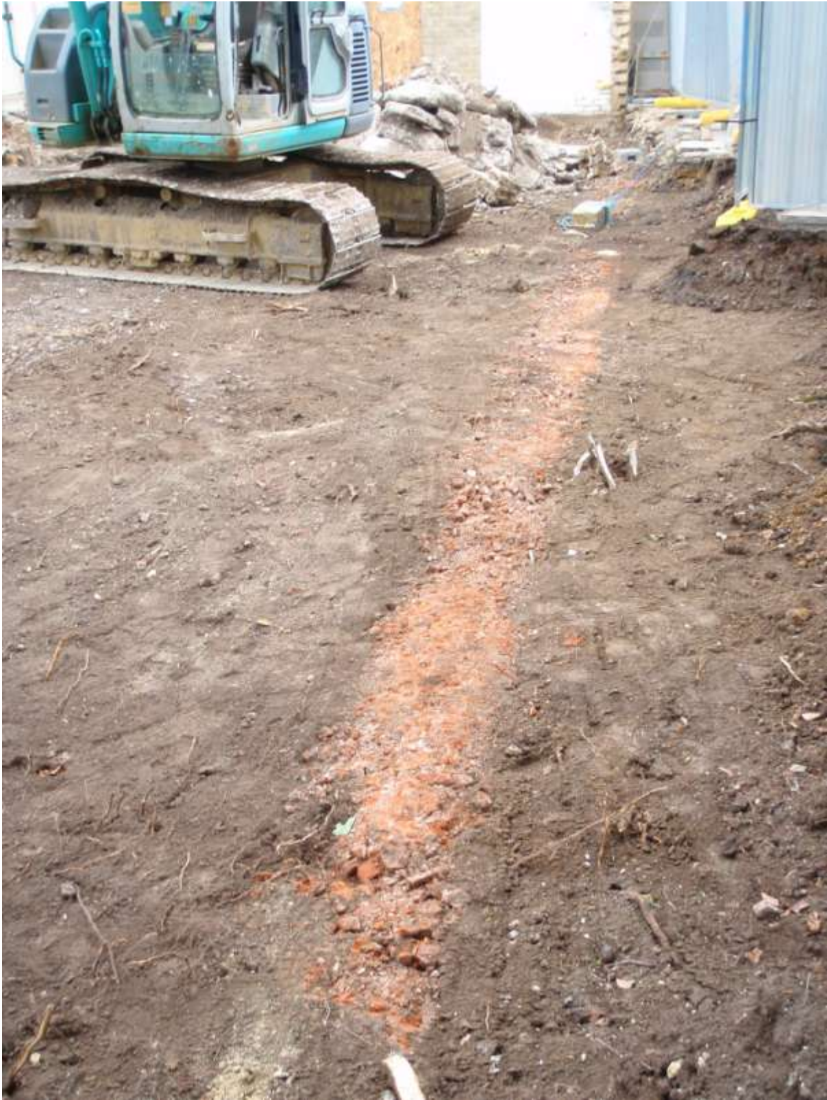
Plate 3. The site showing demolition of garden walls (facing north)
