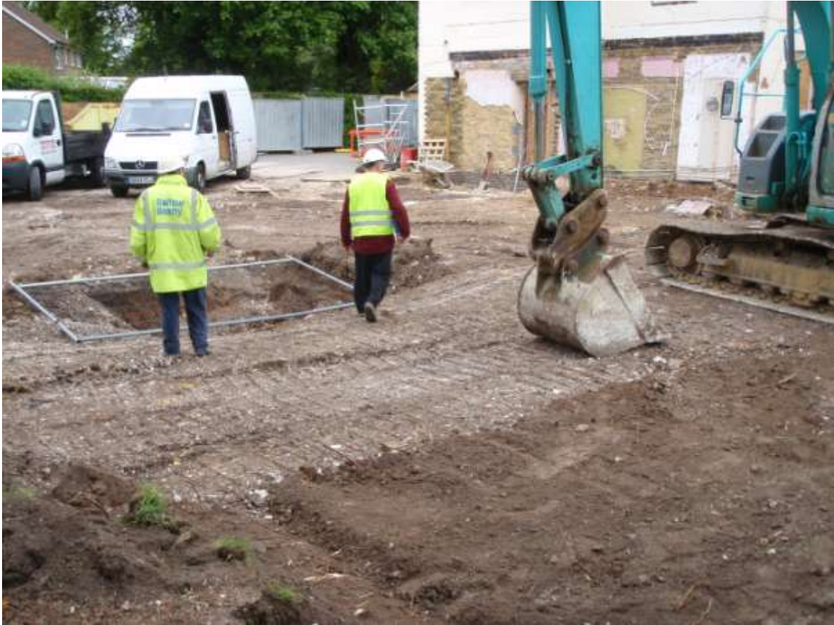
Plate 2. General view of site with area being levelled, facing north-west
