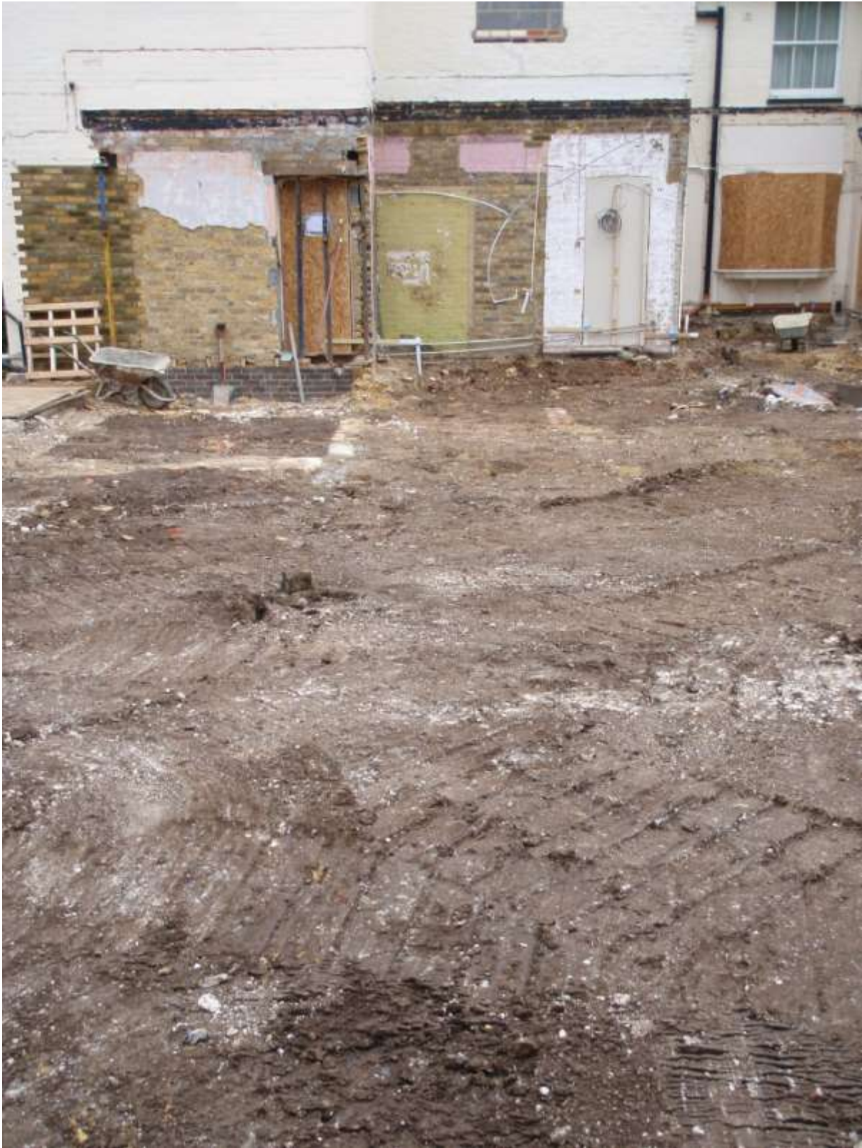
Plate 4. Demolition complete and site levelled (facing north)
